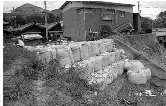
▲洲本川破堤箇所復旧
